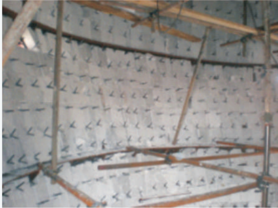
Area of Cement Kiln
